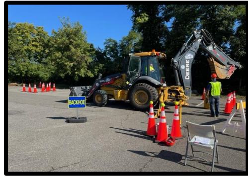
Backhoe being readied for the materials accuracy event
