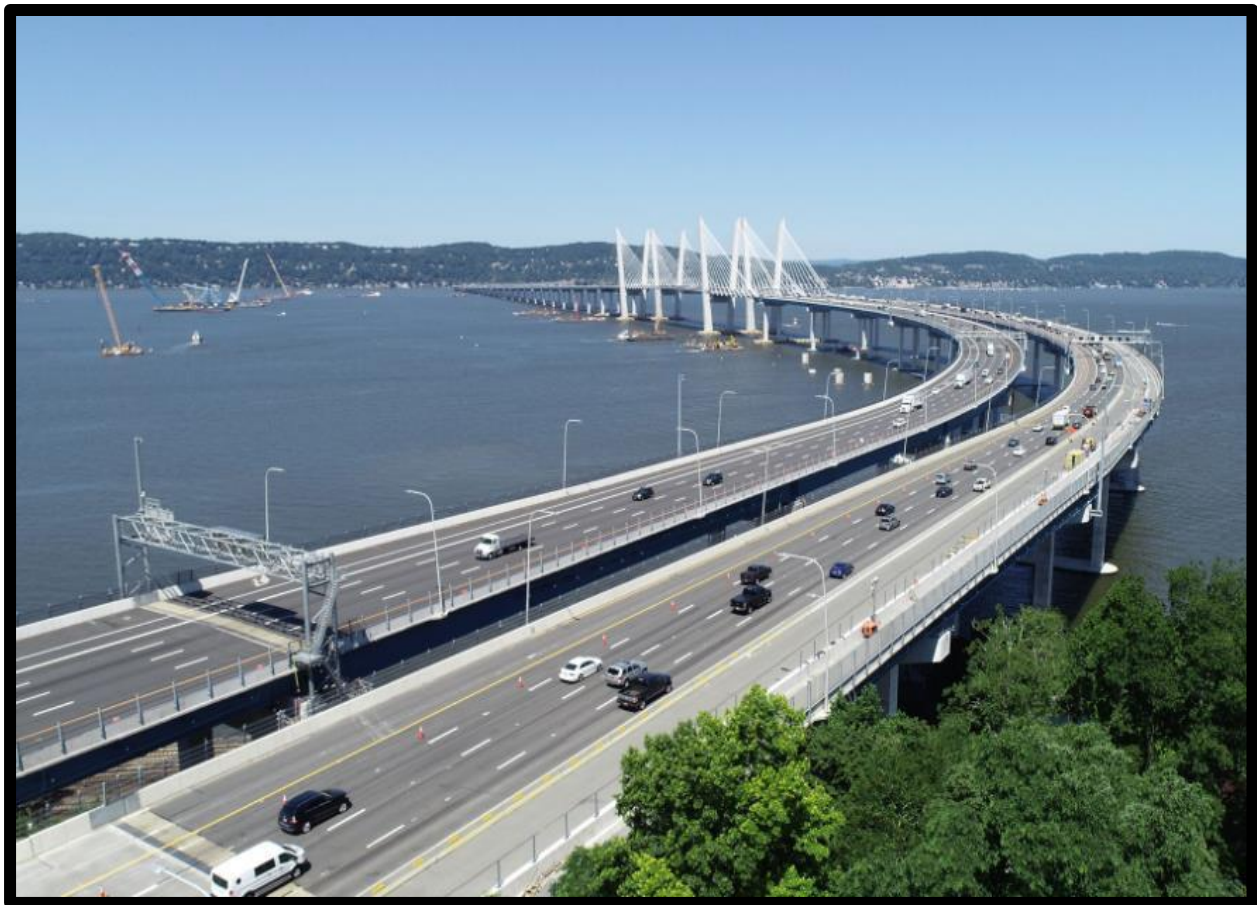
Governor Mario M. Cuomo Bridge viewed from the Westchester County shoreline. Winner of the 2020 Project of the Year Award, over $75 million.
